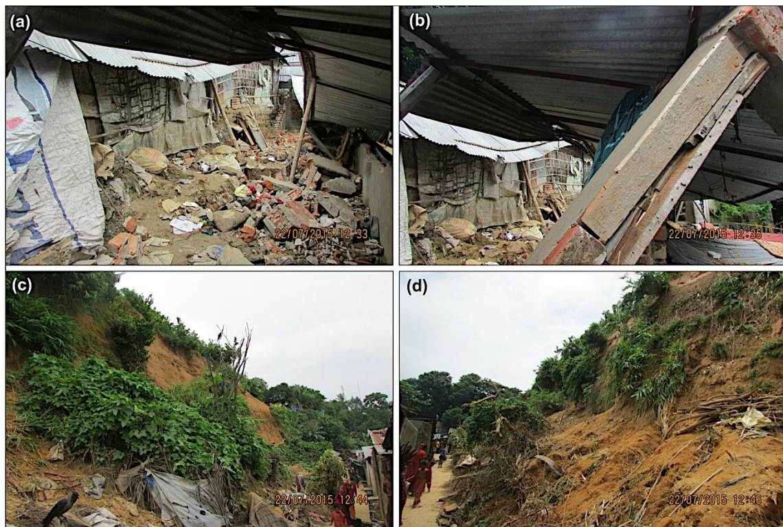
Figure 1 Landslide devastation on 19 July 2015 in Chittagong Metropolitan Area. Source: Fieldwork, July 2015.
