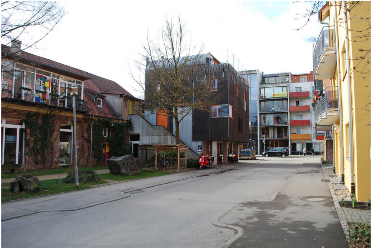
Fig.1 The integration of mixed uses and building ages in the French Quarter.
