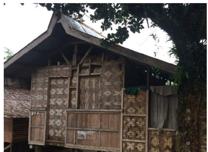
Figure 7: Central roof slope rise for possible wind deflection
