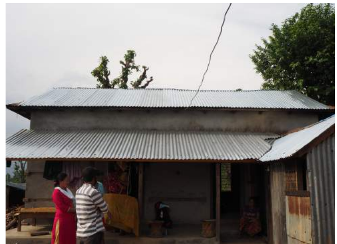
Figure 10: Load-bearing stone masonry, 1.5 storeys
