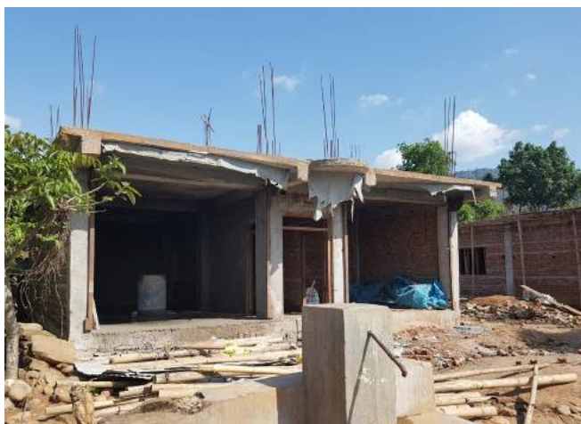
Figure 12: Reinforced concrete frame structure with brick infill walls
