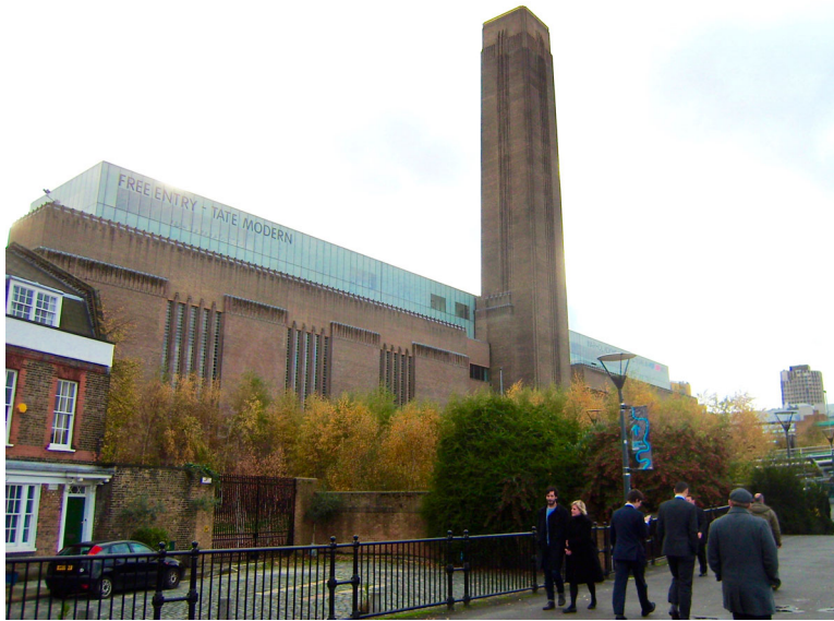
Figure 5. Tate Modern gained the support of the RFAC who recommended against the use of black brick in the alterations given the historic red brick of the structure. Source: Matthew Carmona.
