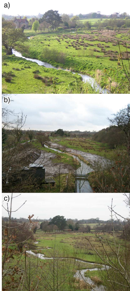
Figure 2. Re-meandered reach of the River Glaven at Hunworth (north Norfolk, UK): (a) in January 2009, prior to the rehabilitation project; (b) after removal of embankments in March 2009; and (c) in December 2010, after recreation of meanders in August. (d) Arc-GIS drawing of the original and re-meandered river channel.
