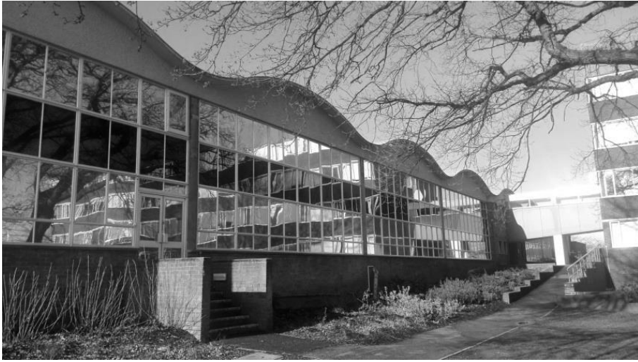
Figure 1. The experimental building.
