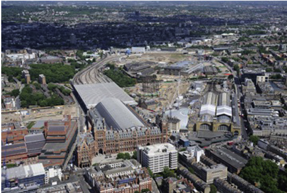
Picture 1. Aerial picture of the King's Cross Central area pre-redevelopment. Source: Arup.
