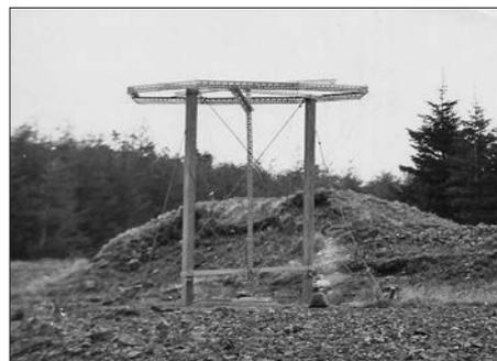
**6** The Hafren experiment. (Left) The equipment trailer on the site labelled Sheep Dip on the Ordnance Survey map. (Right) One of the four monopole conical antennas. The radiating element was a set of wires (not visible in the picture) connected from the upper frame down to a balun transformer on the ground.
