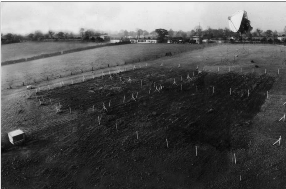
**2** Layout of the equipment looking west, from a montage by RA Porter (1967). The dark area shows the position of the large array. The north-south corner reflector can be seen to the west of the array, in front of the Mk2 radio telescope. The white boxes contained the Geiger counters.
