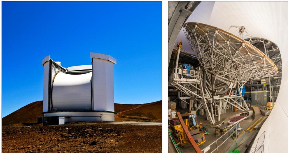
Figure 1. (left) The JCMT in its usual mode of operation with a saddle shaped protective wind blind in place (courtesy of ROE Photolabs) (right) Inside the enclosure showing the wind blind in front of the JCMT dish.
