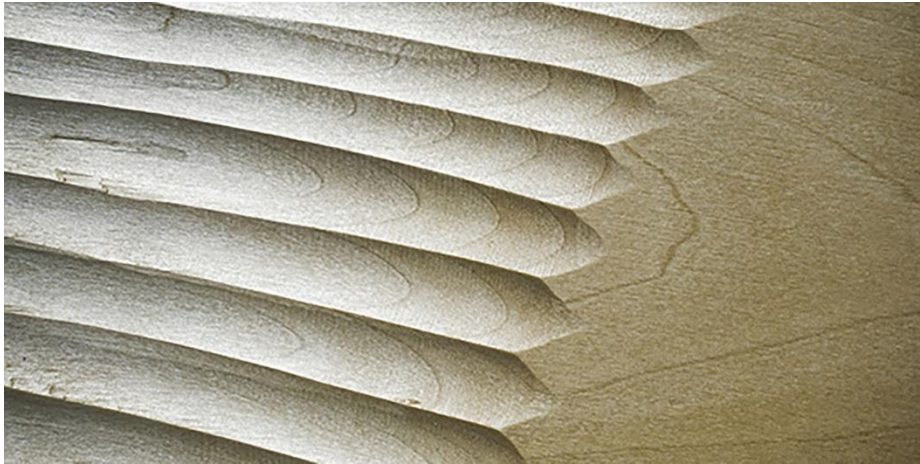
Fig. 10. The training process allows to tune the fabrication system to a specific set of tools and type of wood to explore design opportunities that would become evident only in the fabrication stage.
