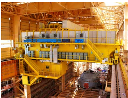
(a) Box girder crane in operation
