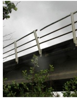
(a) Waiau River Bridge
