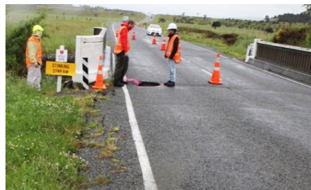
(b) Stinking Stream Bridge SH7
