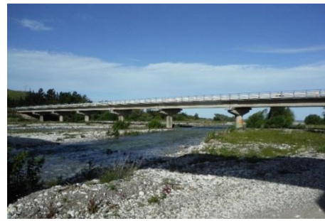
(a) Waima River (Ure) Bridge SH1
