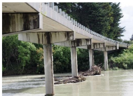
(c) Ferry Bridge, Ferry Road, Spring Creek
