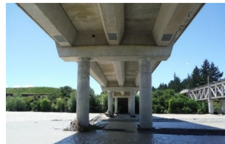
Figure 35: Awatere River Bridge looking north.
