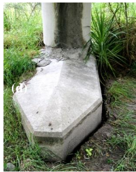
(d) Ground offset with foundation (Mason River Bridge)
