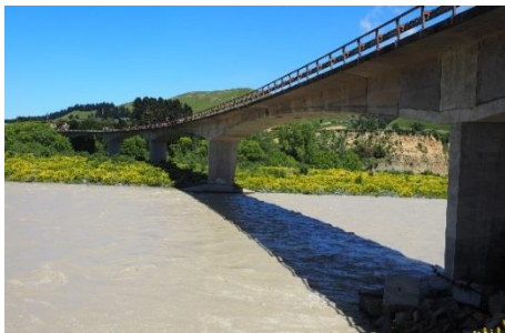
Figure 21: General view of Clarence River Bridge.
