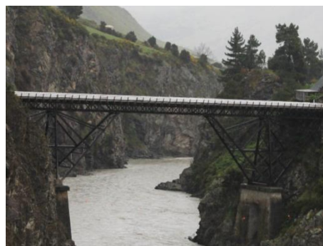
(c) Waiau Ferry Bridge SH7A
