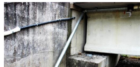
(b) Water pipe (Lower Mason Bridge)
