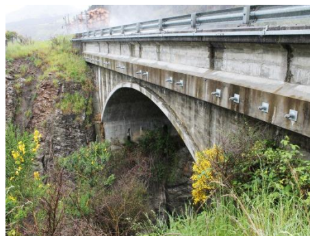
(a) Glenallan Stream Bridge SH7
