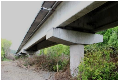
(b) Lower Mason River Bridge - Inland Road
