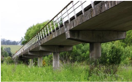
(a) Mason River Bridge – River Road
