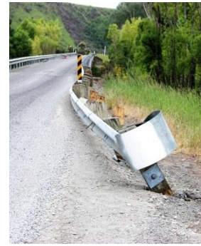
(b) Lower Mason River Bridge
