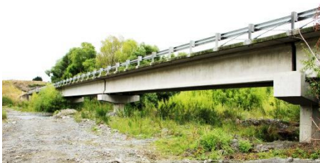
(c) Lottery River Bridge - Inland Road
