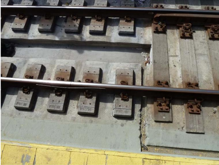
**Figure 26: Section of On-going Construction with Concrete and Wooden Ties.**
