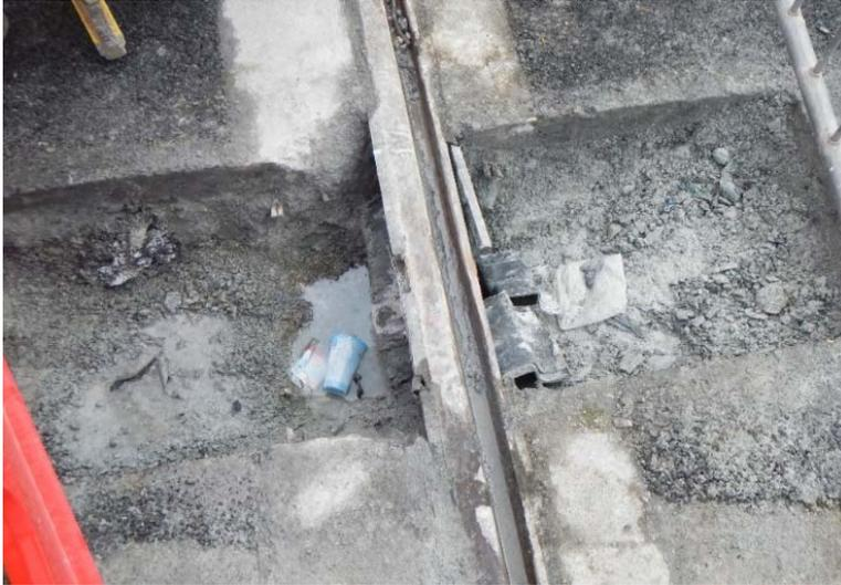
**Figure 10: Broken Rail Rubber Boot on the Rail Requiring Excavation**
