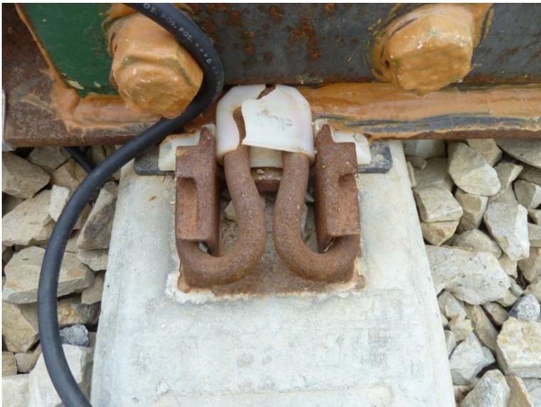
**Figure 9: Cracked Insulation Cap on the Fastener Clip**
