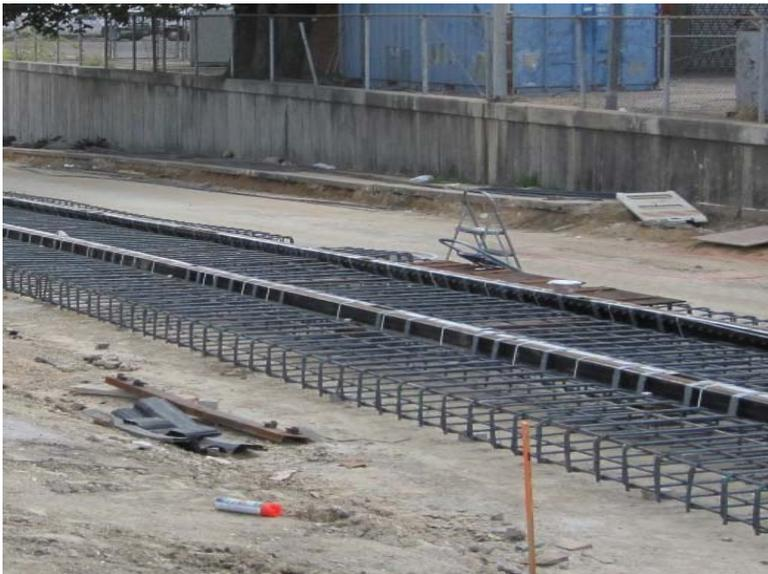
**Figure 22: Steel Reinforcement for the Embedded Slab Track**
