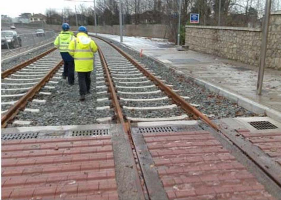
**Figure 29a: Embedded and Ballasted Section**
