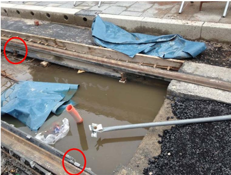
**Figure 11: Missing Insulation at Clips and Missing Rail Boot Overlap**
