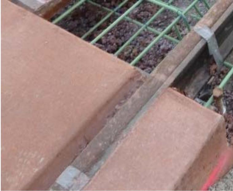
**Figure 43: Tee Rail with Rail Boot and Concrete Groove**
