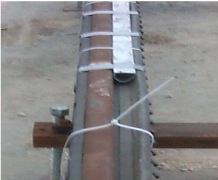
**Figure 42: Tee Rail with Grooved Rail Boot**
