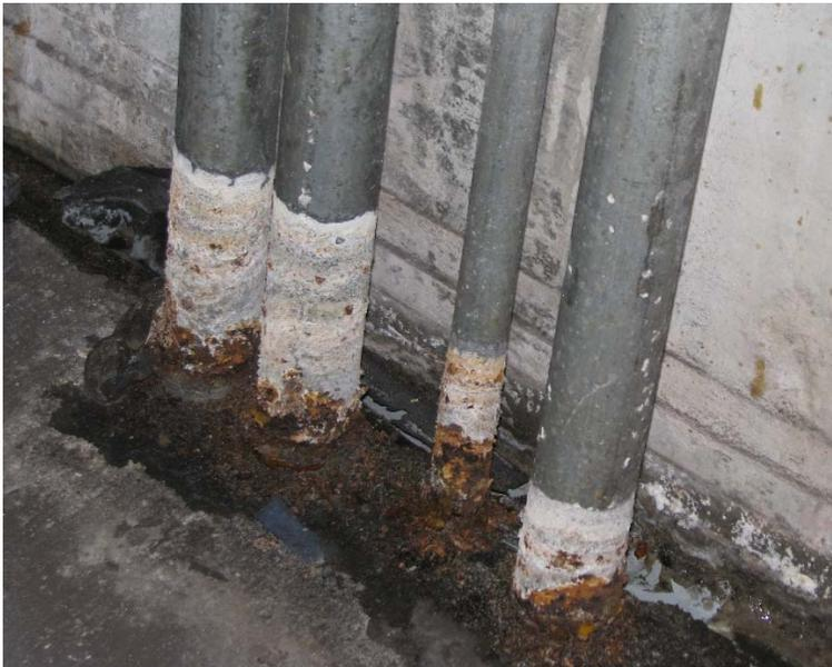
**Figure 29: Corrosion of Pipes at Station Facility (LA METRO)**
