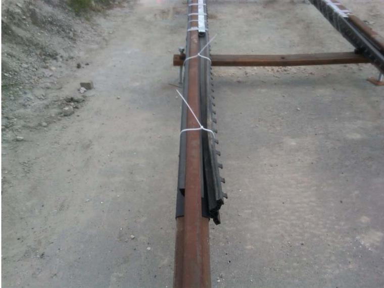
**Figure 21: Section of Flangeway Filler Rail Boot during Construction**
