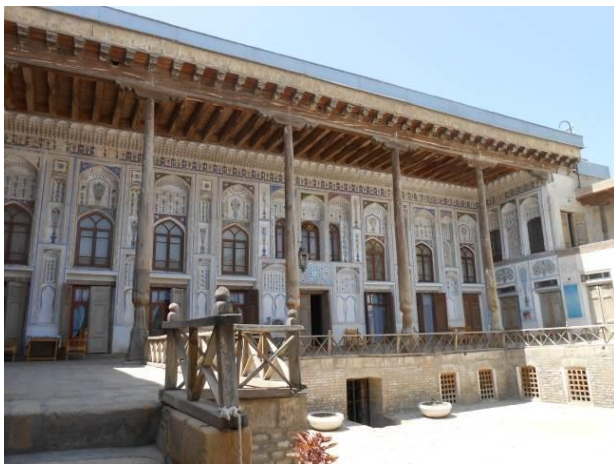
Figure 1. The Jewish House in Bukhara. Traditional Bukharian house with nim-ayvan. © UNESCO field survey project (2013)
