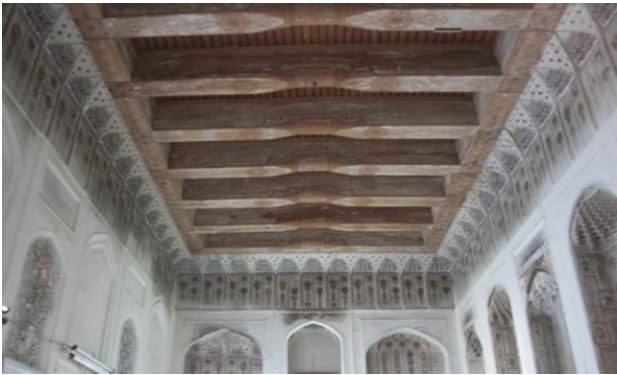
Figure 5. Ceiling beams in a traditional Bukharian house. © UNESCO Field survey project (2013)
