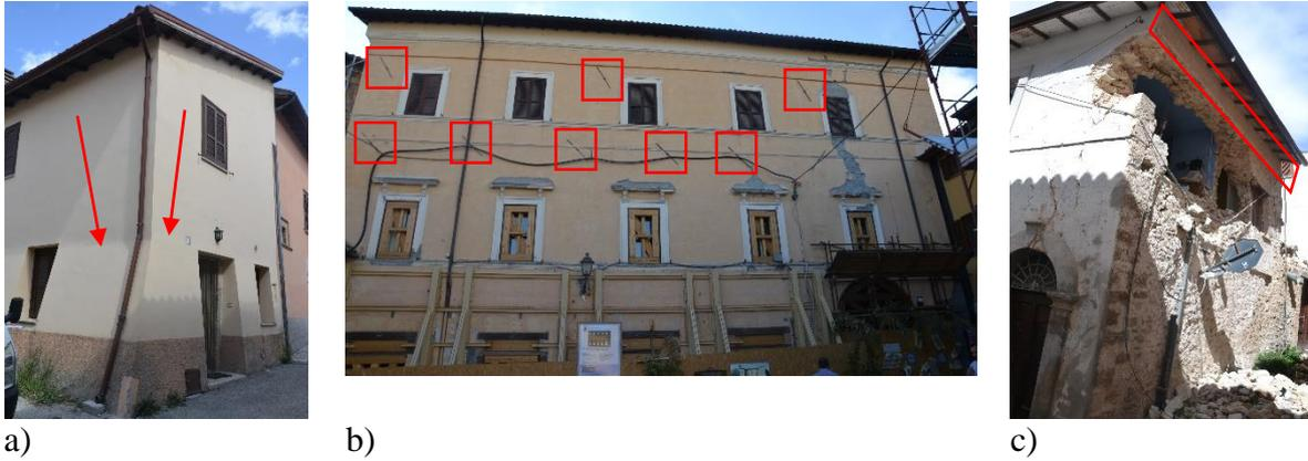
Figure 5: Restraining elements observed in Norcia: a) buttresses, b) ties o c) concrete ring beams
