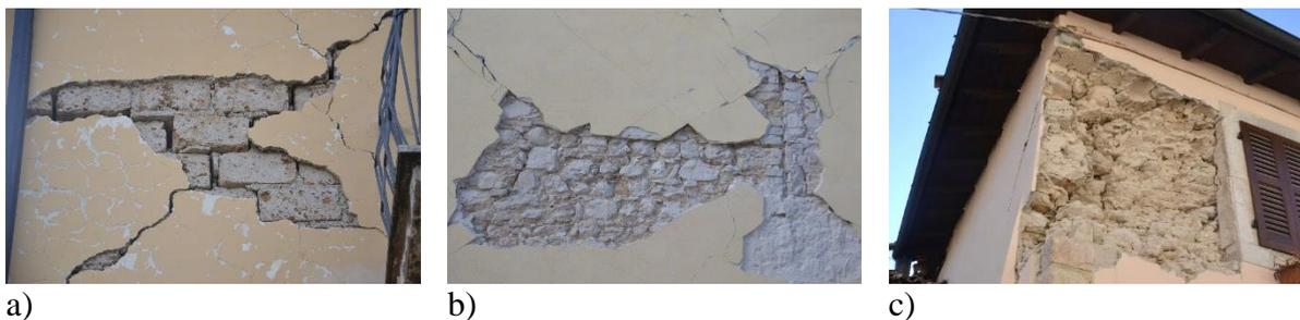
Figure 2: Details of the M1, M2 and M3 masonry types in Norcia
