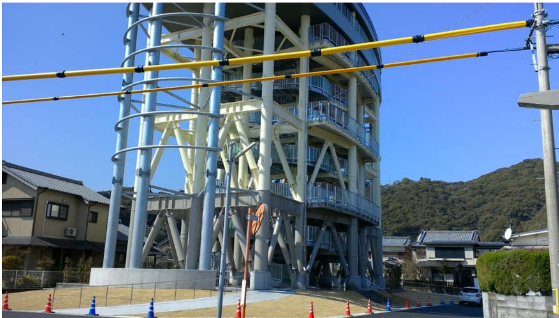
Figure 3. 22-metre high tsunami evacuation tower in Hamamachi Ward in Kuroshio Town.
