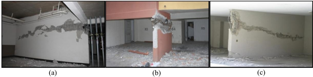
Figure 2. Typical brittle failure in RC walls during the 2010, Maule earthquake: (a) building in Santiago; (b) building in Concepción; and (c) building in Viña del Mar.
