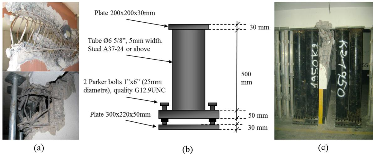
Figure 3. Damage and shoring system: (a) boundary damage and temporary shoring; (b) Yoder pipes and stabilization solution typically used for buildings; and (c) implementation of the stabilization solution at the basement level of a building in Santiago
