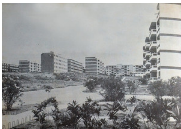
Figure 3 Alamar housing district, Havana, Cuba.
