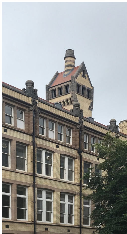
fig.6 Combined ventilation shaft and boiler chimney of the University of Manchester Medical School, designed by Alfred Waterhouse in 1891 (source: James Hopkins)
