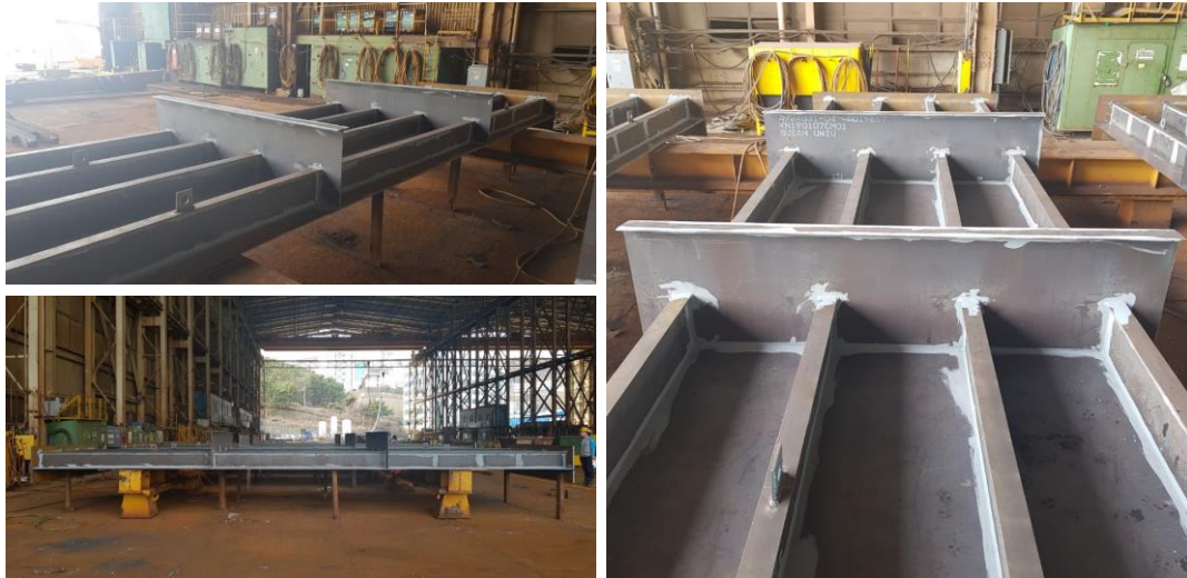
Figure 10. The full-scale steel stiffened plate structure after completion of fabrication in the shipyard.
