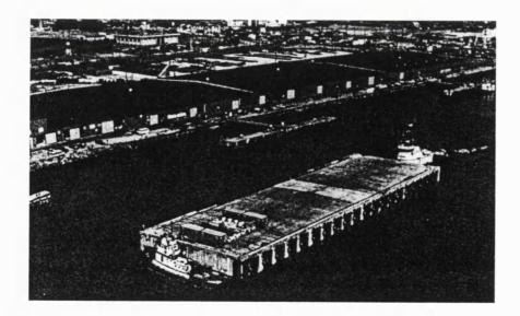
Figure 1.14 Pontoon for Valdez (Alaska) container terminal under tow From construction site (Port of Tacoma) to deployment site [8]
