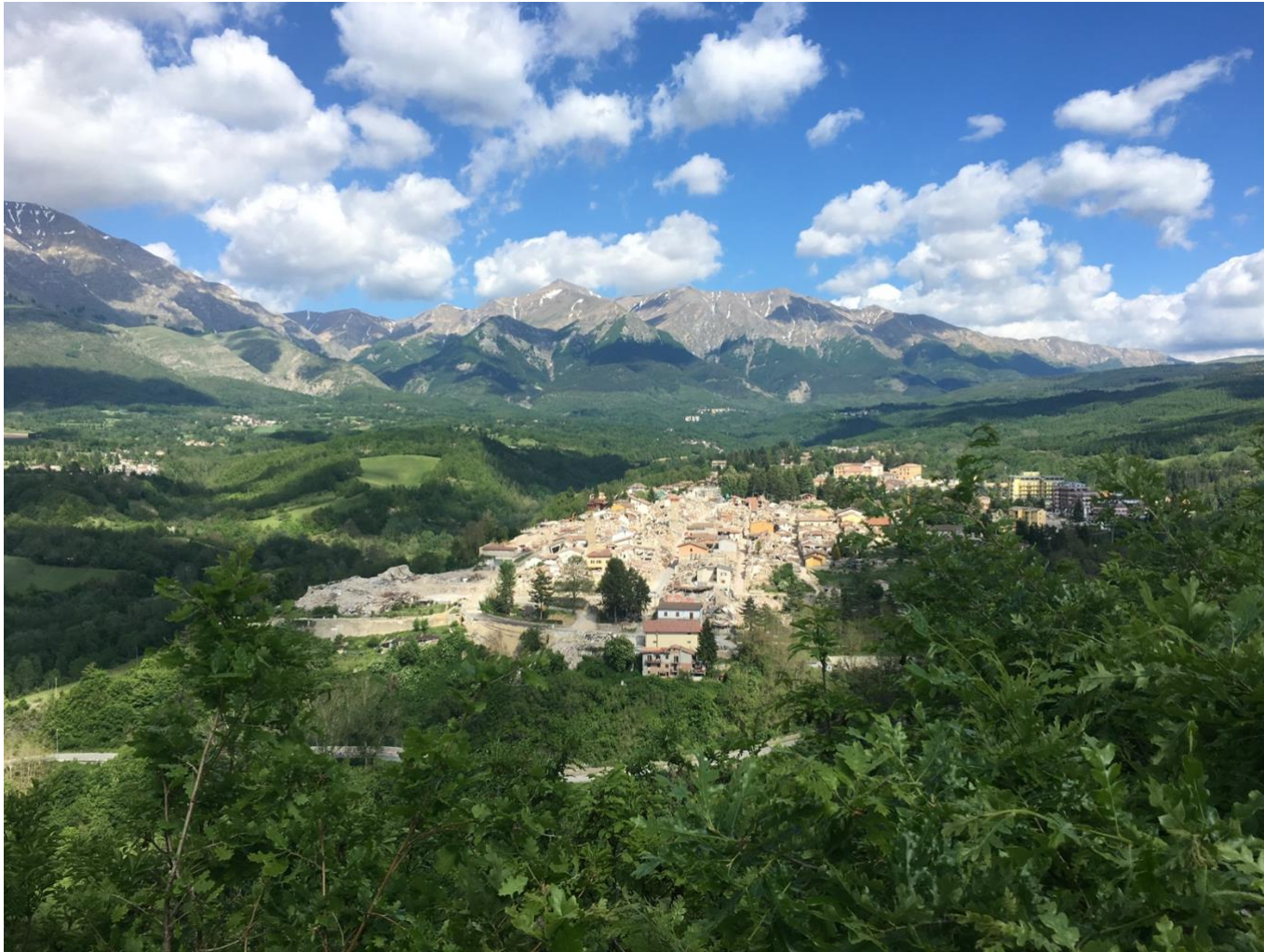
Figure 1.5 The Main Hamlet of Amatrice following the 2016-2017 Central Italy Earthquake Sequence
