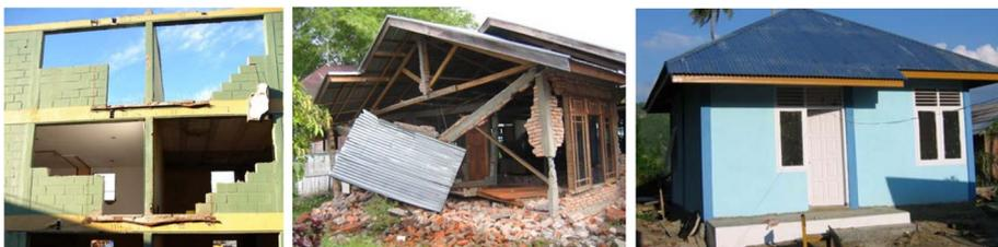
**(a)** Failure of CM walls with no confinement around large openings- 2010 Chile earthquake (Brzev et al. 2010)
