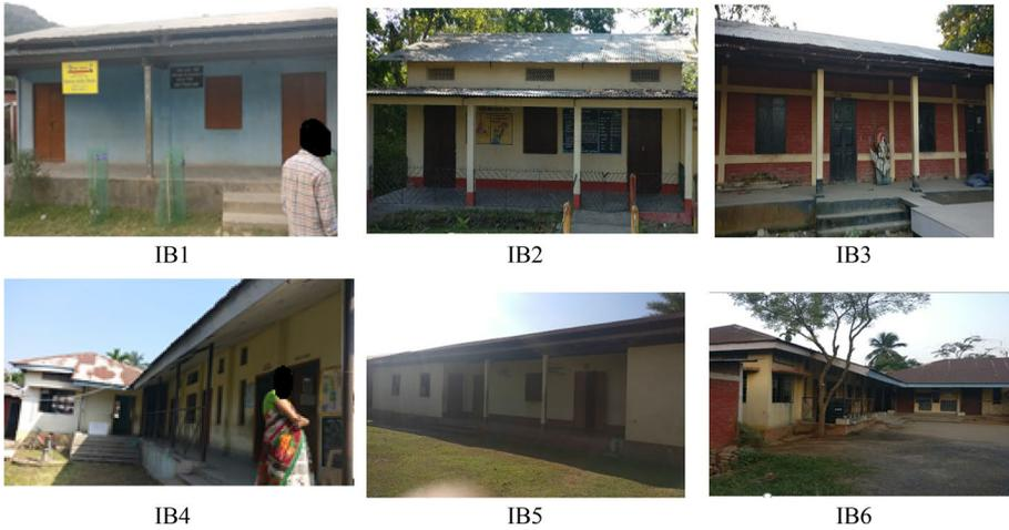
**Fig. 9** Representative buildings in the sample for each of the index buildings: IB1, IB2 and IB3 have simple rectangular plans, while IB4, IB5 and IB6 have irregular plan shape. Other parameters of the IB4-IB6 correspond to IB1-IB3, respectively
