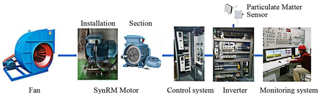
Figure 9: Ventilation system with inverter equipped in metro stations (adapted from [66]).
