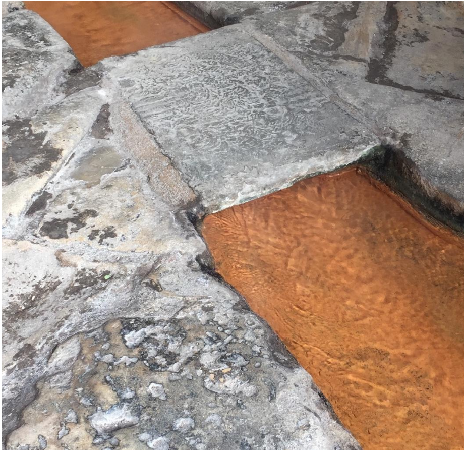
Figure 6.3. Images of the ancient Roman drainage network of the Roman Baths, UK. The images show the orange iron oxide deposits. Images by Tim Walker, 2018.
