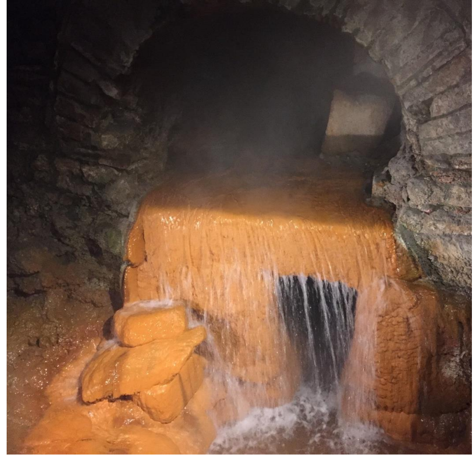
Figure 6.3. Images of the ancient Roman drainage network of the Roman Baths, UK. The images show the orange iron oxide deposits. Images by Tim Walker, 2018.
