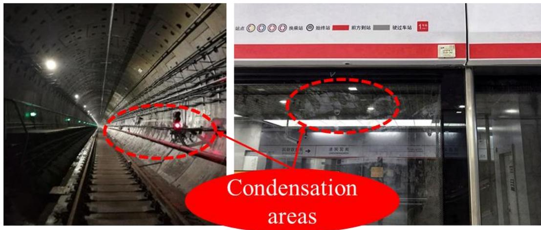
Figure 1. Condensation on tunnel walls and platform doors in an underground station.
