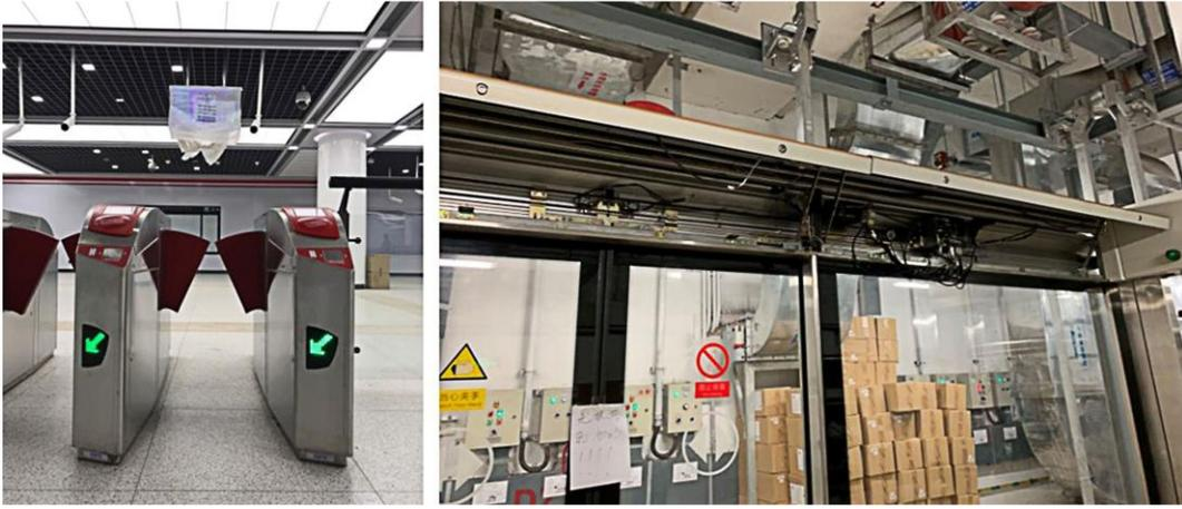
Figure 4. The automatic gate machine and the motor of the PSD system.
