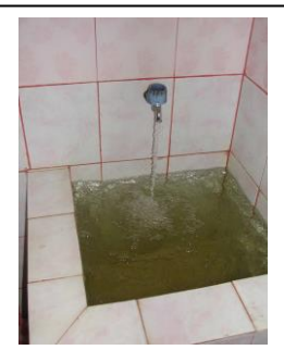
Figures 5.4, 5.5, 5.6, and 5.7 A typical of water installation made by individual households. Residents installed new boreholes or wells, electric jet pumps, elevated water tanks, and plumbing systems for water circulation inside the houses. As the quality of groundwater was not good, they purchased mineral water for drinking purposes. Source: field survey 2002.
