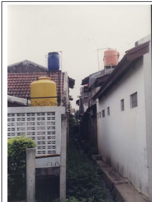
Figures 5.4, 5.5, 5.6, and 5.7 A typical of water installation made by individual households. Residents installed new boreholes or wells, electric jet pumps, elevated water tanks, and plumbing systems for water circulation inside the houses. As the quality of groundwater was not good, they purchased mineral water for drinking purposes. Source: field survey 2002.
