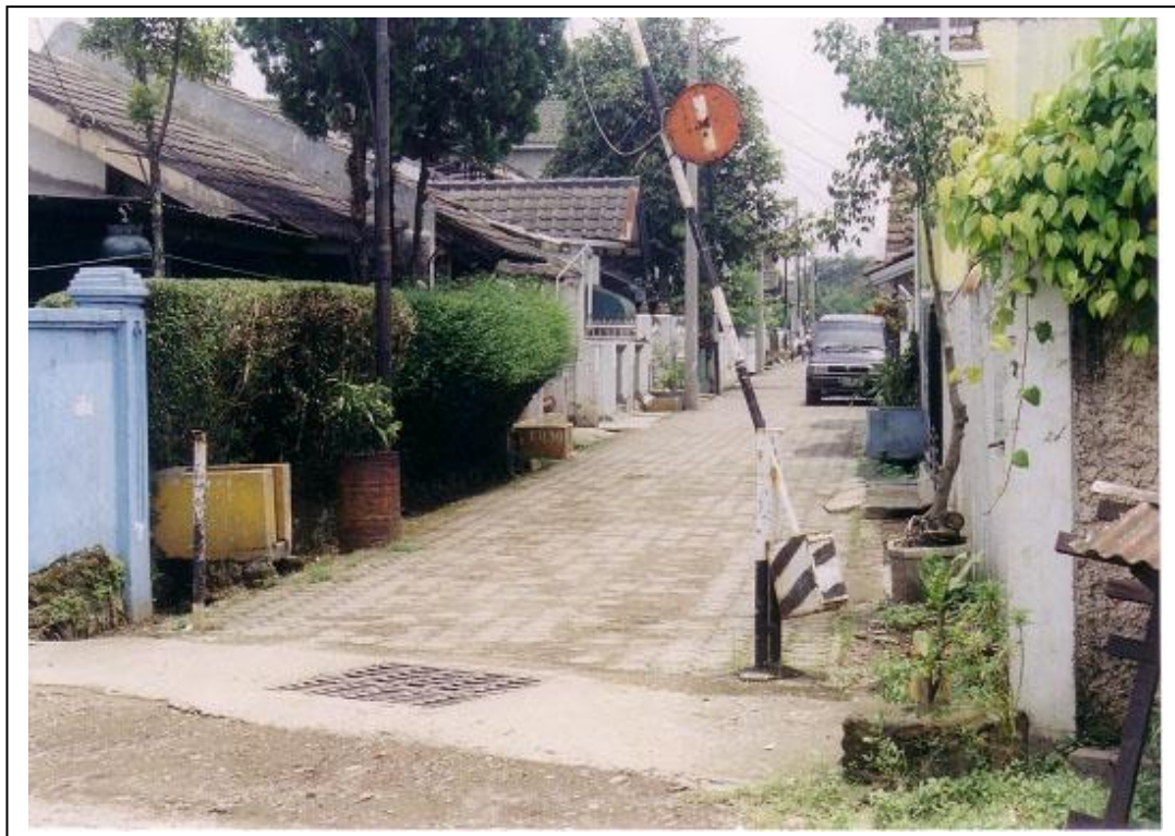
Figure 5.25 An example of road improvement by the residents. Residents preferred paving-blocks to tarmac for the improvement. A portal fence was installed to prevent heavy vehicles from entering, and this was also used as a security barrier during the night, as robbery was common in the MRRA. Source: field survey 2002 .
