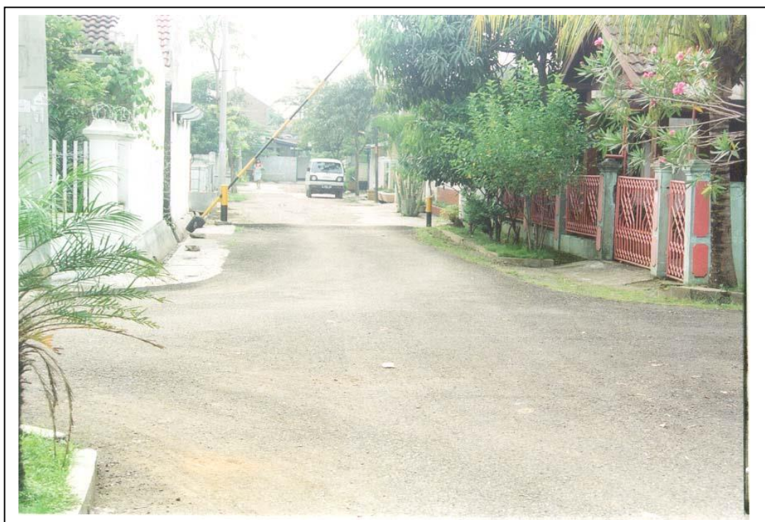
Figure 5.26 Another example of collective road improvement. Residents of this neighbourhood preferred tarmac to other materials and portal fences were installed for security reasons. A distinctive mark under the portal fence (at the edge of the tarmac), which is a hump, distinguished the start of the neighbouring community that was not involved during the mutual self-help action. Source: field survey 2002 .
