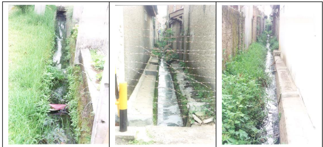
Figures 5.8, 5.9, and 5.10. A typical combination of drainage-sewerage. It was common that rain/grey water could not flow freely because of high sedimentation, weeds, and even garbage blocking the ditch. Households arranged regular collective work either by contributing labour or hiring somebody else to make the drainage-sewerage function. The position of the ditch behind the two rows of houses prevented it from spreading bad odour to the front sides of the houses. Source: field survey 2002.
