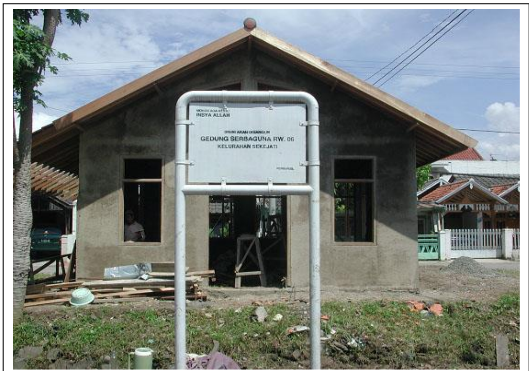
Figure 5.22 An example of a multipurpose building development. After more than fifteen years the community group (an RW) decided to construct this building. The lack of free land for a plot compelled them to erect the building on an area that was previously a tiny park. Source: field survey 2002.
