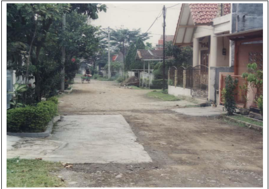
Figures 5.27 and 5.28 The absence of collective road improvement. When this happened, households improved the road in front of their houses individually. The main purpose was for sheltering their cars while they were out of the garages. Source: field survey 2002.
