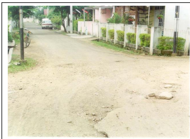
Figure 5.29 Road improvements. The community in this neighbourhood had recently finished its road improvements and used tarmac (in the background). However, it neglected part of the road in the foreground, considering that this was an access to another neighbourhood. Source: field survey 2002.
