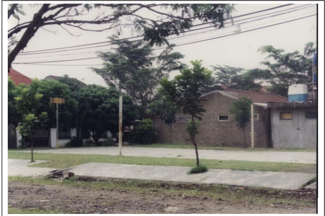
Figure 5.17 An example of a combined volley-basketball court. Residents set up this facility using mutual self-help. However, maintenance apparently stopped, for the basketball board was broken and the road in the foreground was left damaged. The land was initially a vacant site that was given to the project by the developer. Source: field survey 2002.
