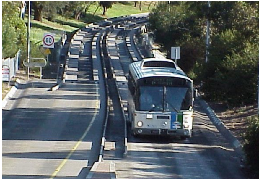
Fig. 38 ▲ Adelaide’s so-called O-Bahn system uses mechanical guides.
