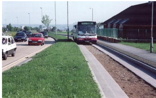
Fig. 16 ▲ ◀ Not paving the centre of the BRT lane can produce substantial cost savings and reduce noise.
