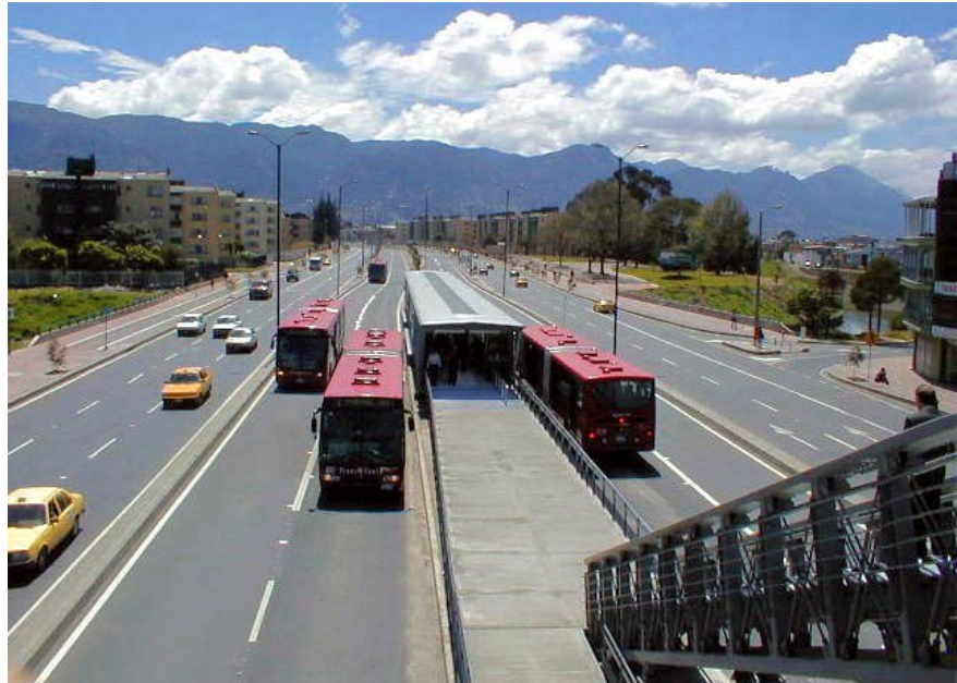
Fig. 19 ▲ Busway located in the centre median. Photo courtesy of TransMilenio SA, Municipality of Bogotá, Colombia
