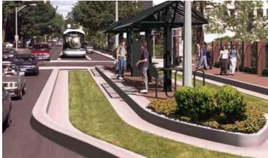
Fig. 16 ▲ ◀ Not paving the centre of the BRT lane can produce substantial cost savings and reduce noise.
