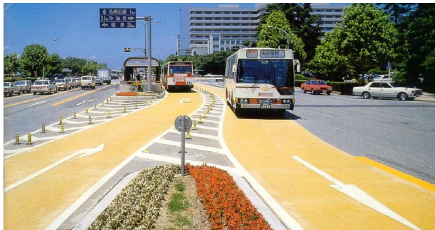
Fig. 17 ▼ Coloured lanes raise the profile of the busways, as can be seen in Rouen, France and Nagoya, Japan.
