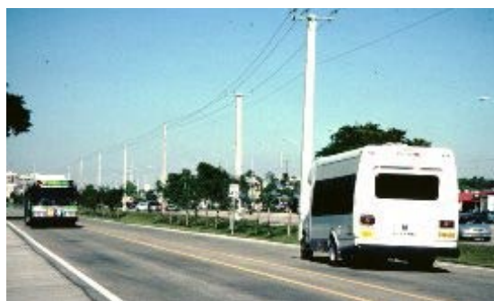
Fig. 21 ◀ Both busway lanes located on one side of the road in Miami, USA. US Federal Transit Administration
