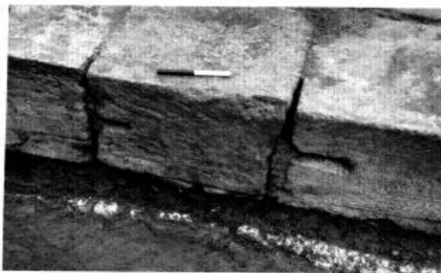
Fig 40 Peter's Hill; detail of limestone blocks in the massive foundation. Note Lewis holes. The dark material beneath the blocks was a backfill timber slot, beneath which the first chalk raft is visible. (Scale 2 x 0.10m)
