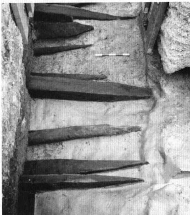
(a) layer of sharpened timbers, laid on the natural clay.
