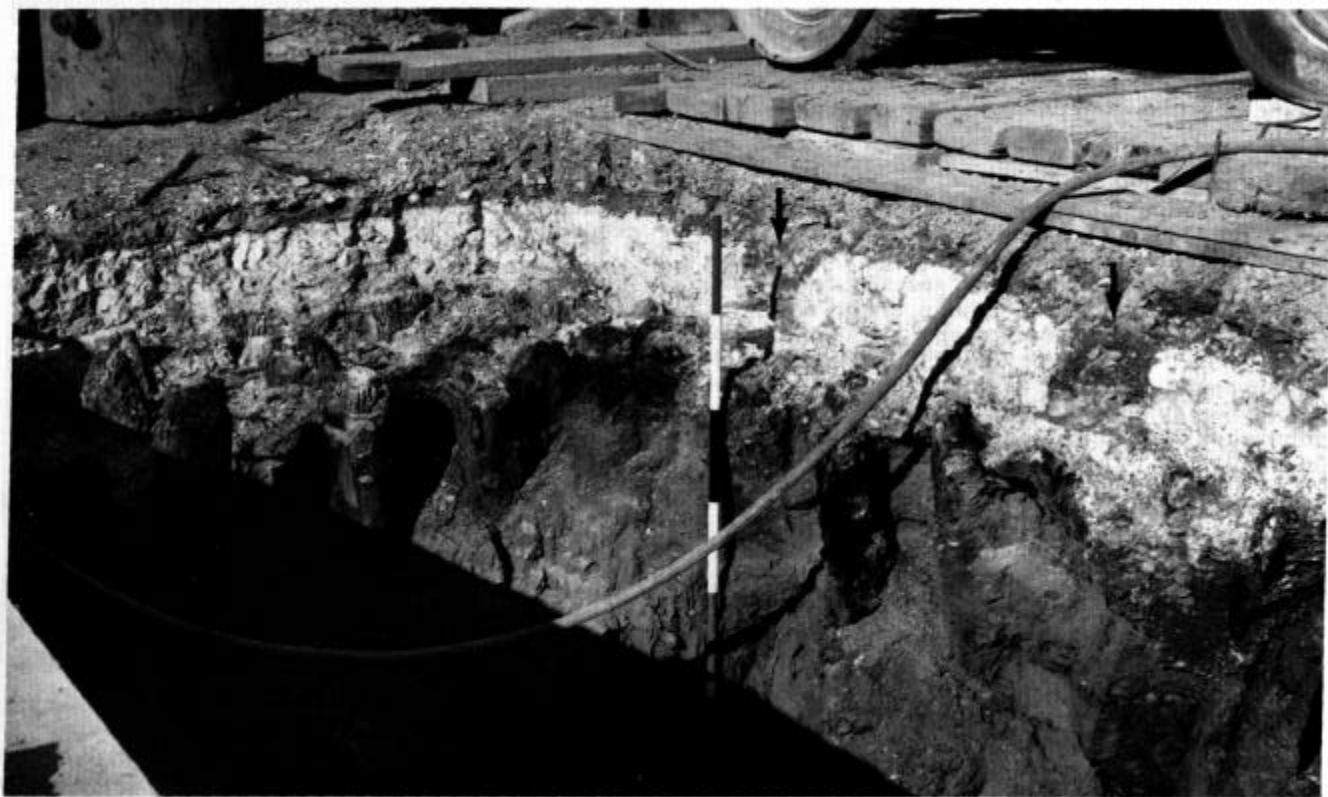
Fig 17 Salvation Army Headquarters; timber piles and chalk raft exposed during building works. Arrows indicate possible slots in the second chalk raft: evidence of a horizontal timber framework. (Scale 6 x 1')
