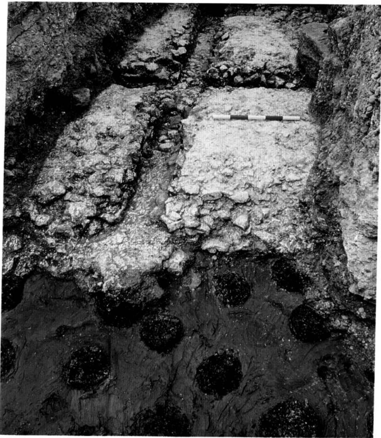
Plate 1 Peter's Hill; timber slots and the second chalk raft (looking west). Note the sharp profiles of the 'slots' and the undisturbed first chalk raft, which formed their base. The timbers were placed directly upon the first raft, with the second raft packed around them. The oak pile support for the first raft is visible in the foreground. (Scale 5 x 0.10m)
