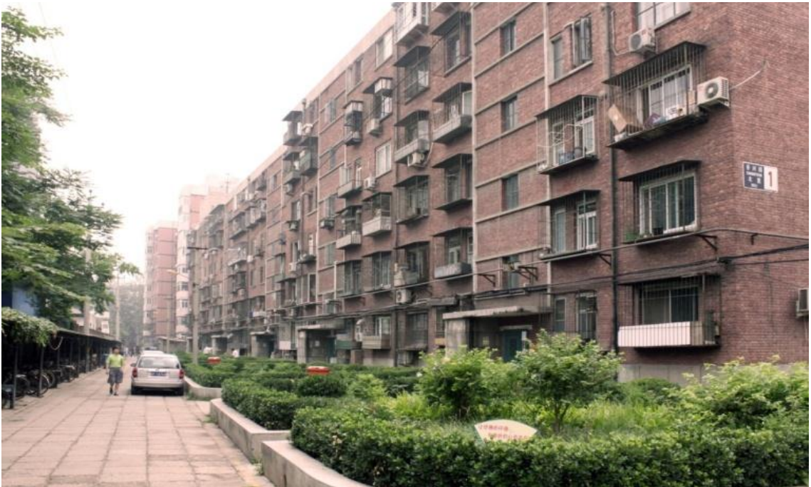
Figure 80: Workers' community. The image shows the six-story tall loufang in the workers' community. This type of luofang , with concrete and brick structure, is the commonest type constructed in the 1970s and 1980s. The loufang in the image was the oldest workers' housing in the paper mill community. (Photo the author, 16 June, 2009).
