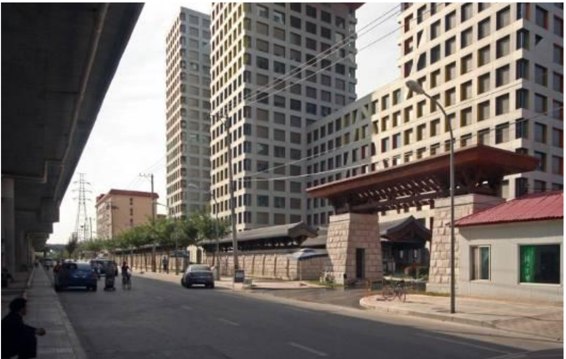
Figure 28: New wall and gate constructed to enclose Linked hybrid. (Photo the author, 14 September, 2009).
