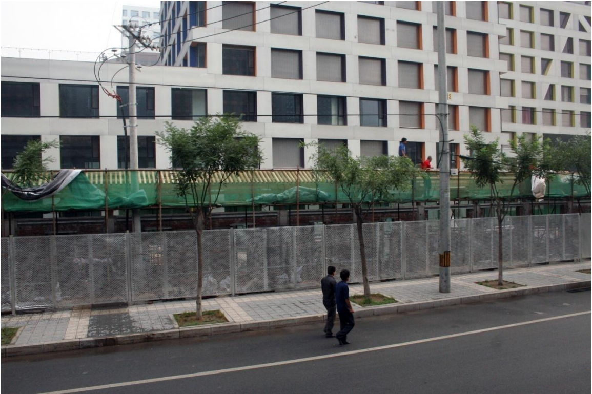
Figure 27: Construction of the wall. (Photo the author, 13 July, 2009).
