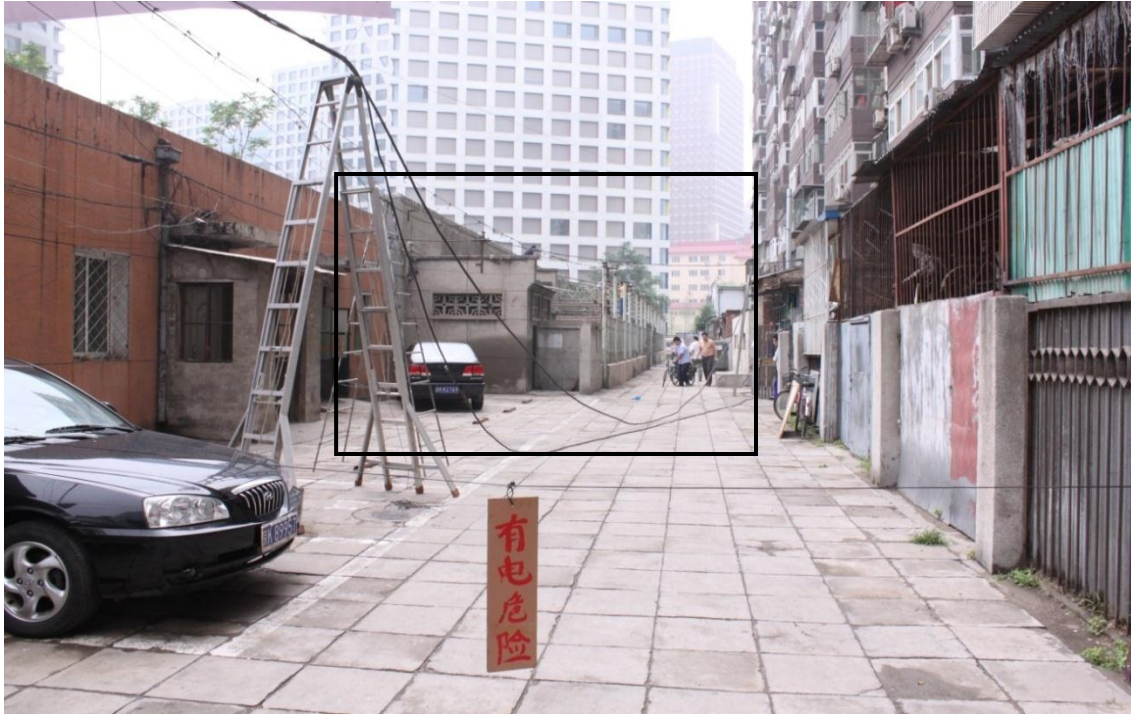
Figure 40: Bicycle canopy before renovation. The old bicycle storage structure is highlighted in the image. Only part of it had a roof. (Photo the author, 16 June, 2009).
