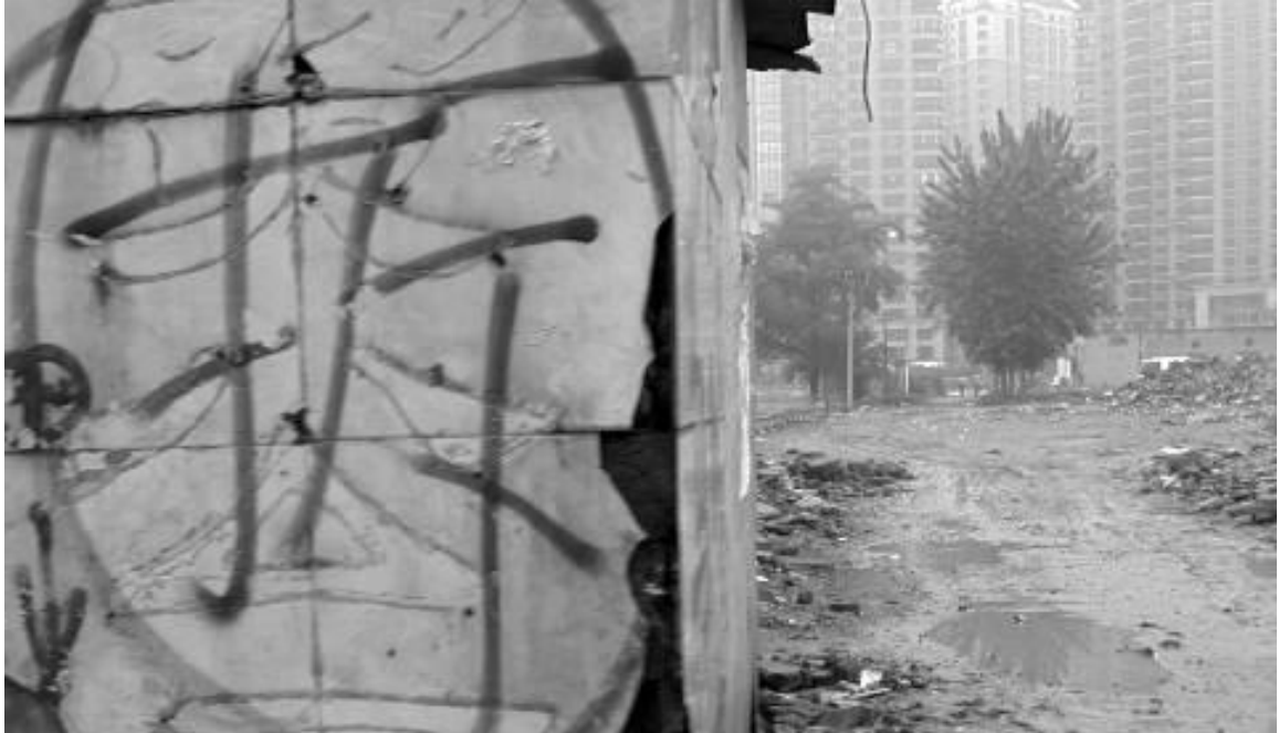
Figure 54: The sign of chai on a ready-to-be-demolished structure in the workers' community. The structure is a restaurant at the entrance of the workers' single-story dormitory at the south-western end of the development property shared by Linked Hybrid. After an interview with Li Hu, he recommended that we see the demolition site. (Photo the author, 14 June, 2008).
