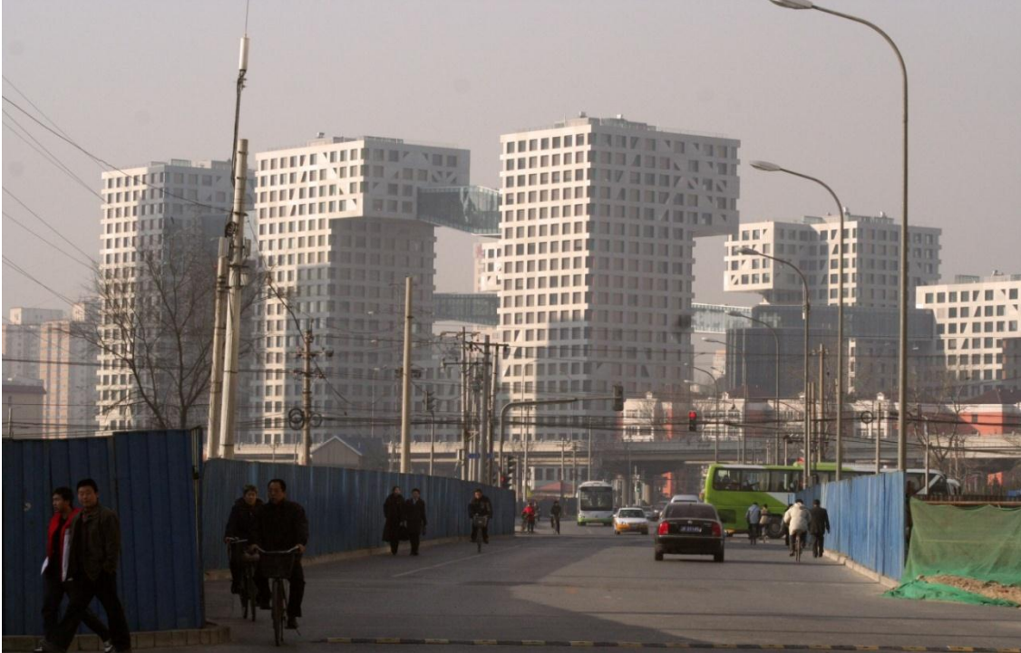
Figure 5: Beijing Linked Hybrid under construction. (Photo the author, 14 December, 2008).
