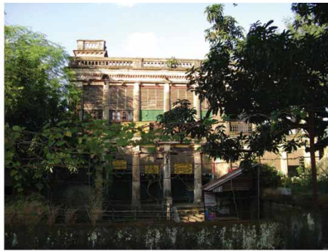
Figure 24. a. ground and first-floor plans, section; b. view from outer court: Baithak-khanna of the Chakrabarty residence, Suri.
