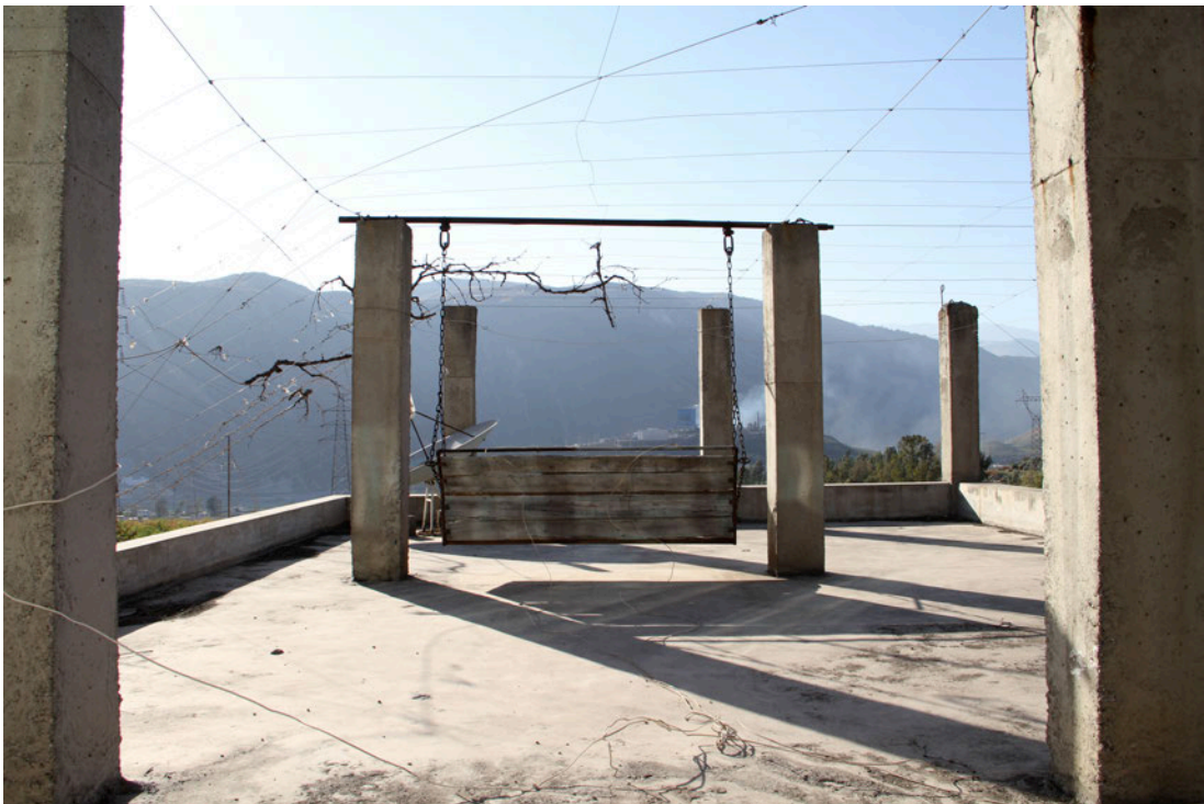
Figure 11: Concrete pillars on the roof of Mr Xu's house leave the possibility for adding an additional floor in the future. Meanwhile the space is used for an improvised rocking chair.
