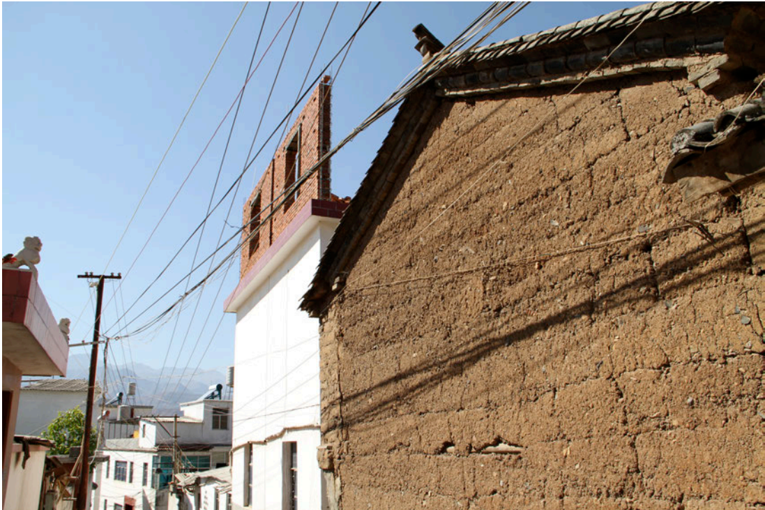
Figure 5: One of the few remaining soil houses in the village-in-the-city. A number of village-in-the-city homes can also be seen in the background.
