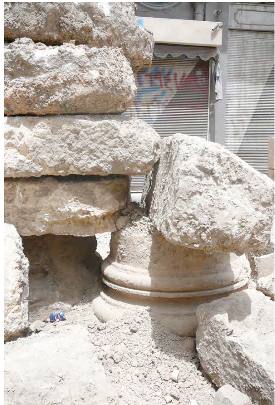
12 - destroyed Roman columns
