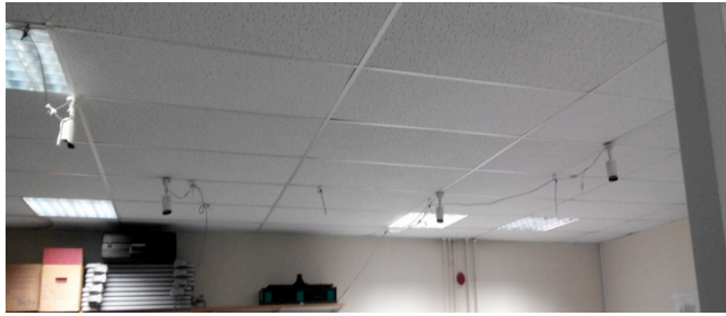
Figure 8. Four cameras connected in a U-shape.
