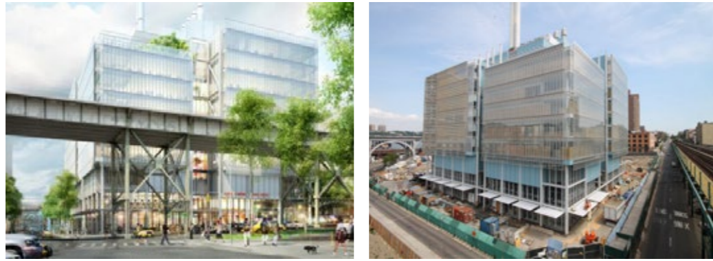
Columbia University Manhattanville campus, Science Center: rendering (left), and under construction (right). Images courtesy Renzo Piano Building Workshop (left), Columbia University 2015 (right)
