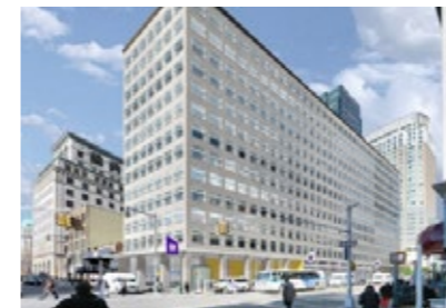
NYU: new facilities at Jay Street, Brooklyn. Image courtesy NYU
