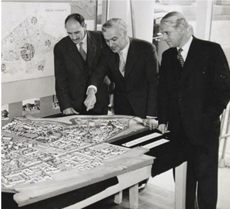
Figure 2.8: Planners (from left to right) Percy Johnson-Marshall, LW Lane and Hubert Bennett examine further plans for the reconstruction of Stepney-Poplar (1955), UEA 237/PJM/LCC/E/2.3.2 .
