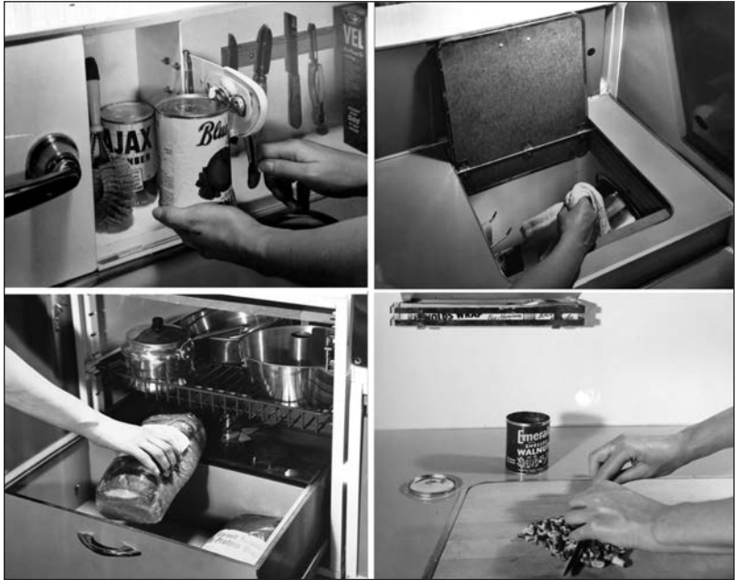
FIG. 5 Samples of the Cornell Kitchen's built-in features (clockwise from top left): can opener at sink center; towel storage at sink center; cutting board at mix center; and breadbox at mix center. All are photos of the kitchen installed at the Housing Research Center Laboratory, 1954. (Source: NYSC, Box 77, folder 12.)
