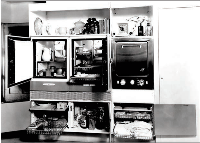
FIG. 10 Oven-refrigerator unit, 1954. Note pullout trays in fridge. (Source: CHES, Box 11, folder 18.)
