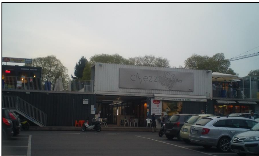
Figure 4.5. The shopping centre “ Cavezzo 5.9” constructed using containers. At the end of 2016, the containers have been dismantled and donated to the population affected by the Central Italy earthquake in August 2016. Photo taken during the field trip in April 2014.
