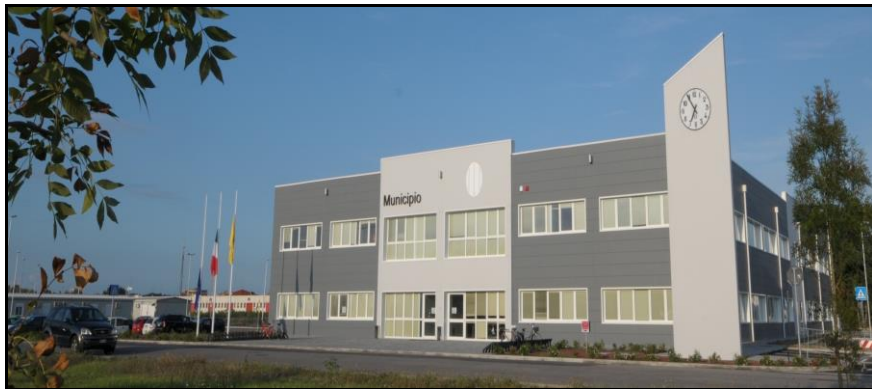
Figure 4.3. The new building of the city hall in Mirandola. Besides to it, a new school for the town has been built. Source: Comune di Mirandola website
