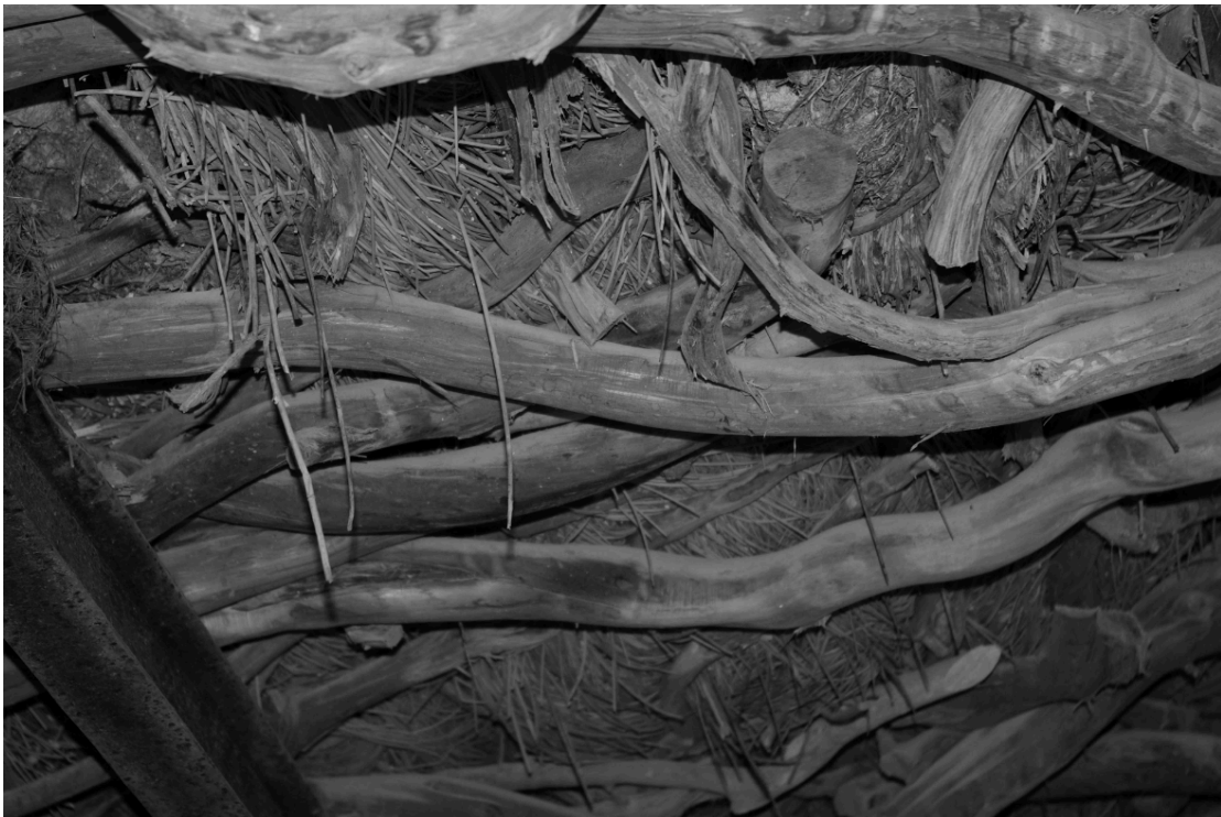
Figure 10. Wooden roof beams of juniper ( Juniperus phoenicea ) in an abandoned building
