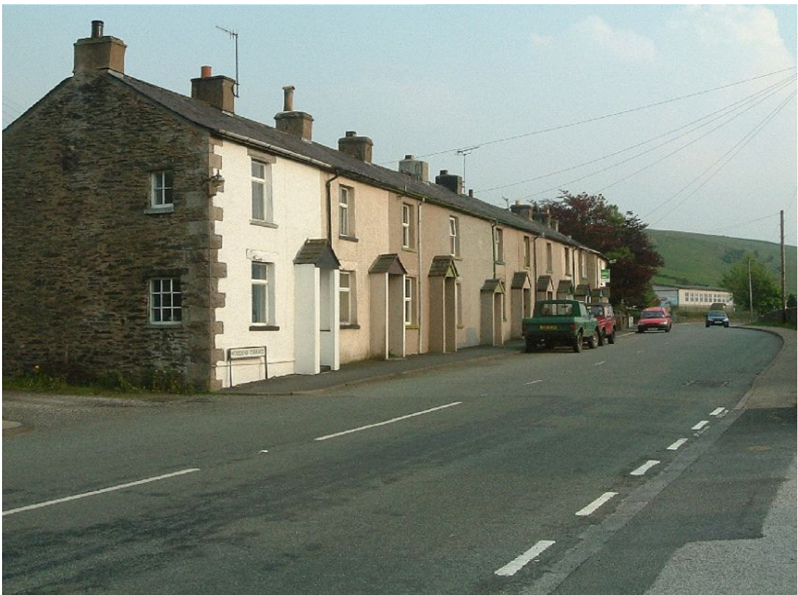
Figure 5: Tebay, Cumbria (CA10 3): The Standardised Ratio for Terraced Houses is 136.
