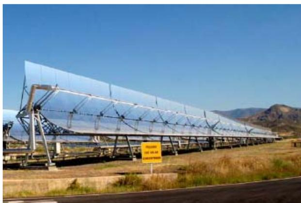
**Figure 2.15** Medium-concentrating solar collectors - parabolic trough collectors at PSA, Spain (source: <http://www.psa.es/webeng/instalaciones/parabolicos.php>).
