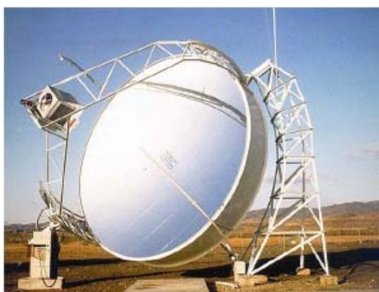
**Figure 2.16** High-concentrating solar collectors - parabolic dish at PSA, Spain (source: <http://www.psa.es/webeng/instalaciones/discos.php>).
