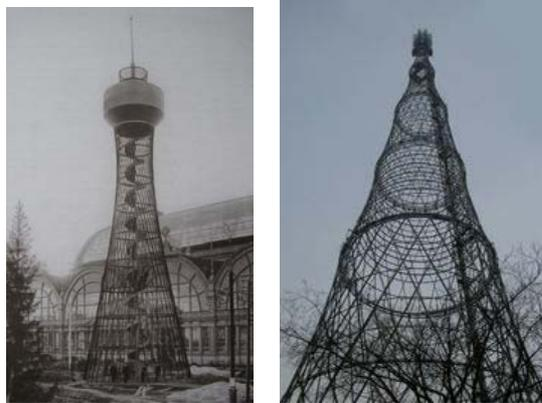
Figure 13. The world's first hyperboloid water tower, All-Russian Exposition, Nizhny Novgorod, Russia, 1896 (Images from Wikipedia, <http://en.wikipedia.org/>)
