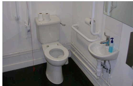
Figure 8: Unisex Cubicle with poor colour contrast between fixtures & fittings. Photo; VivaCity 2020: 2005
