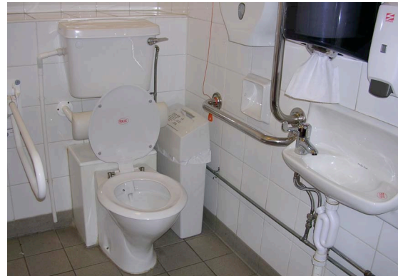
Figure 7: Flush handle fitted on wrong side of WC pan, also too high for some users. Photo; VivaCity 2020: 2005
