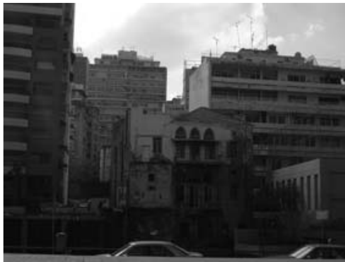
Figure 1: .The façade of a Central Hall type house with its wide arcade opening and red tiled roof, as it stands today in Central Beirut.
