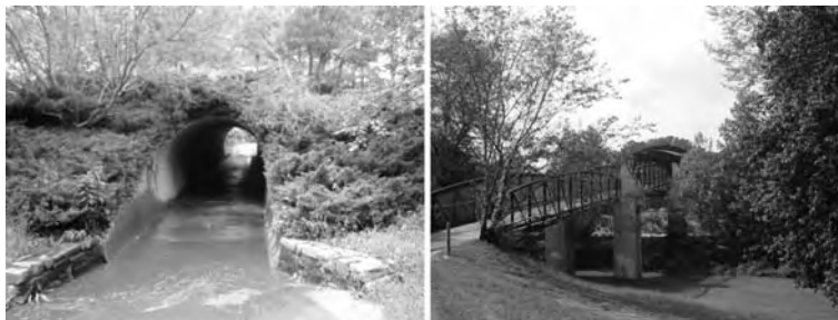
Figure 4.3. View of a Typical Cart Path Tunnel and Bridge Crossing
