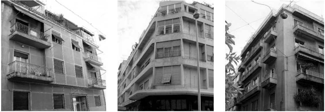
Figure45 Typical multi-storey residential buildings [Grigoratos and Sfiriou,2006]
