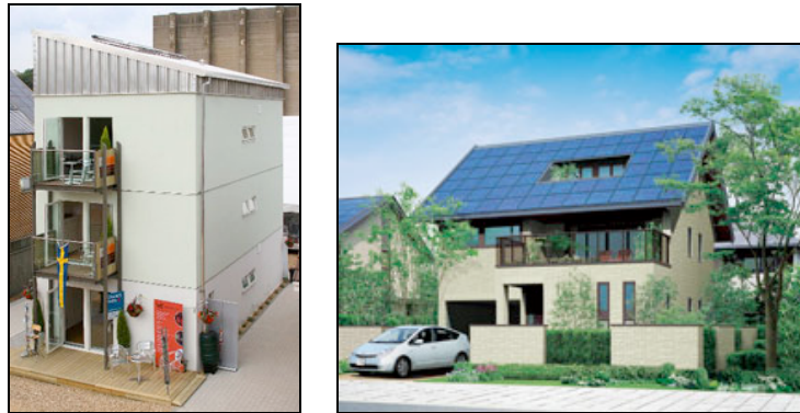
Figure 10: Houses by ecoTECH (UK) and Sekisui House (Japan)
