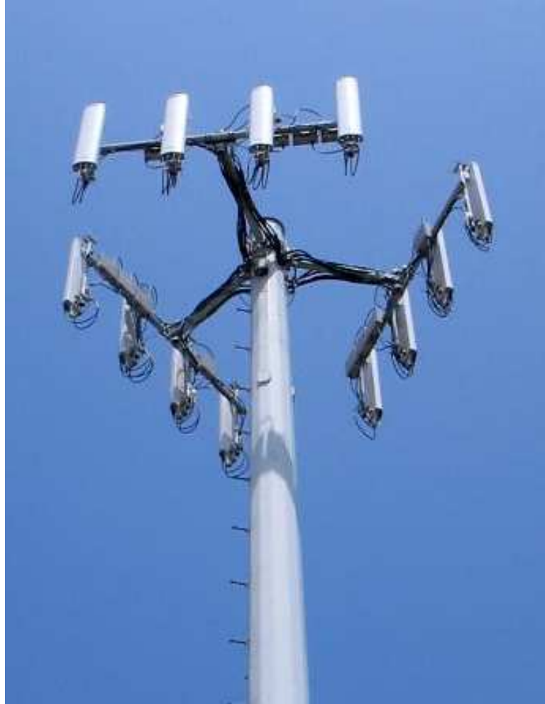
Figure 1.2: Multiple antennas at a base station of a cellular system. Photo obtained from [14].
