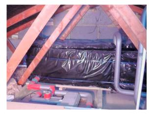
Figure 2: a) insulation missing above ceiling near eaves b) lack of insulation beneath cold water tank.
