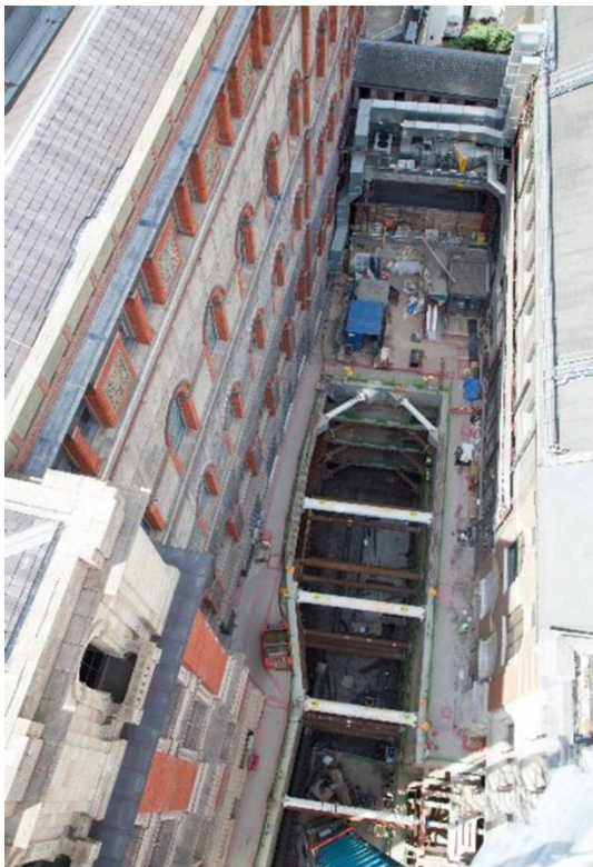
Figure 5.10: The dog leg basement excavation area (courtesy of Arup Geotechnics)
